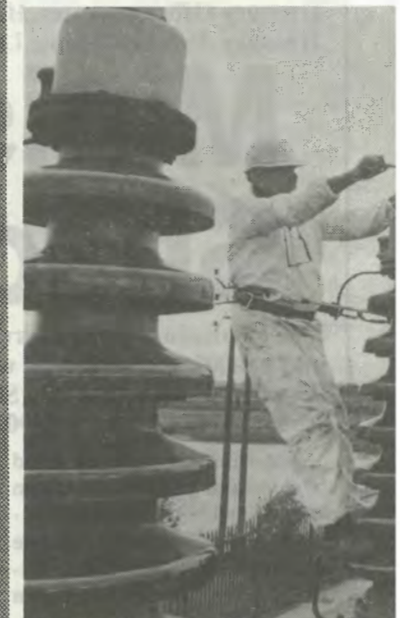
Above: Chargehand Electrical F on high voltage bushings at Seala
