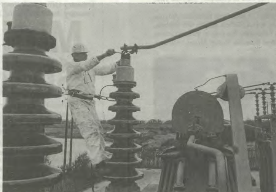
Above: Chargehand Electrical Fitter Ian Harris checks primary connections on high voltage bushings at Sealand Sub-station.
